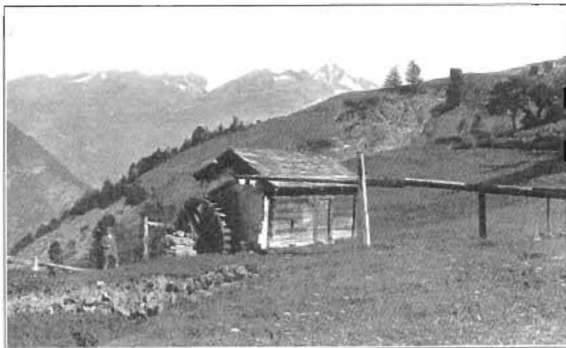
Fig. 8—The grist mill at Visperterminen for producing entire rye flour and meal
